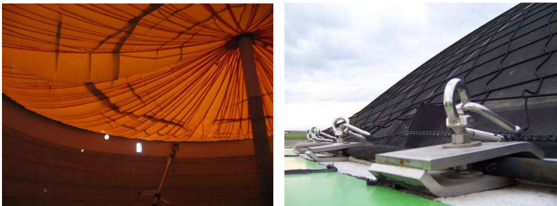
Figure 7.27 Digester cover of gas tight membrane, seen from the inside of the tank -left (AGRINZ 2006); Digester cover of gas tight membrane, outfitted in exterior with expansion net -right (RUTZ 2006)
