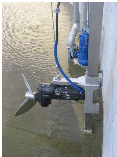
Figure 7.22 Submersible motor propeller stirrer (AGRINZ 2006)
