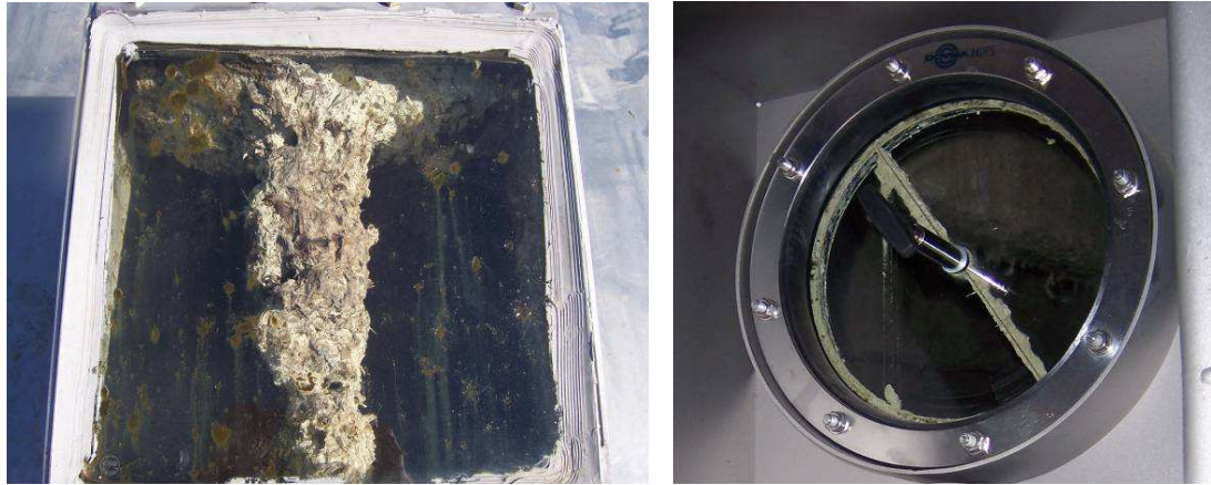
Figure 7.29 Elementary sulphur, resulted from biological desulphurization inside the digester (RUTZ 2007)
