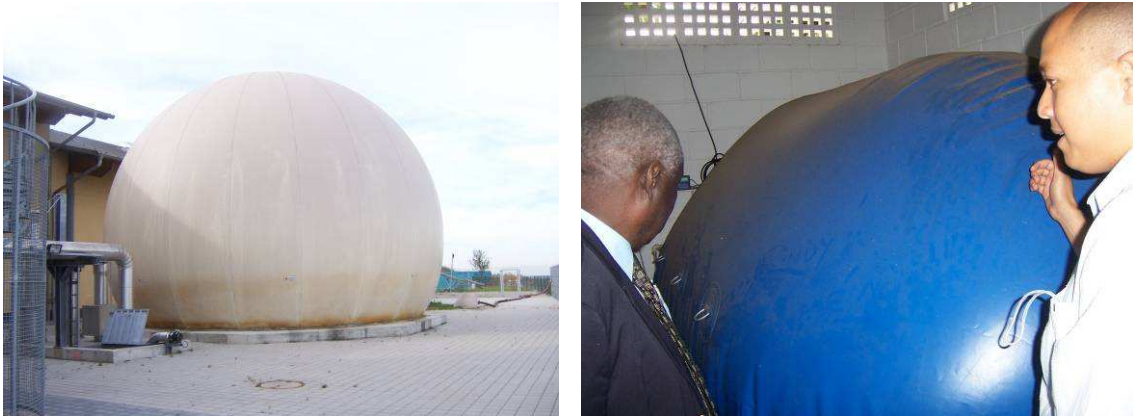
Figure 7.26 External low pressure gas storage tanks (RUTZ 2007)
