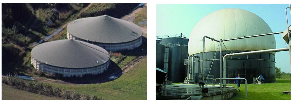
Figure 7.33 Membrane covered storage tanks (DANISH BIOGAS ASSOCIATION 2008)
